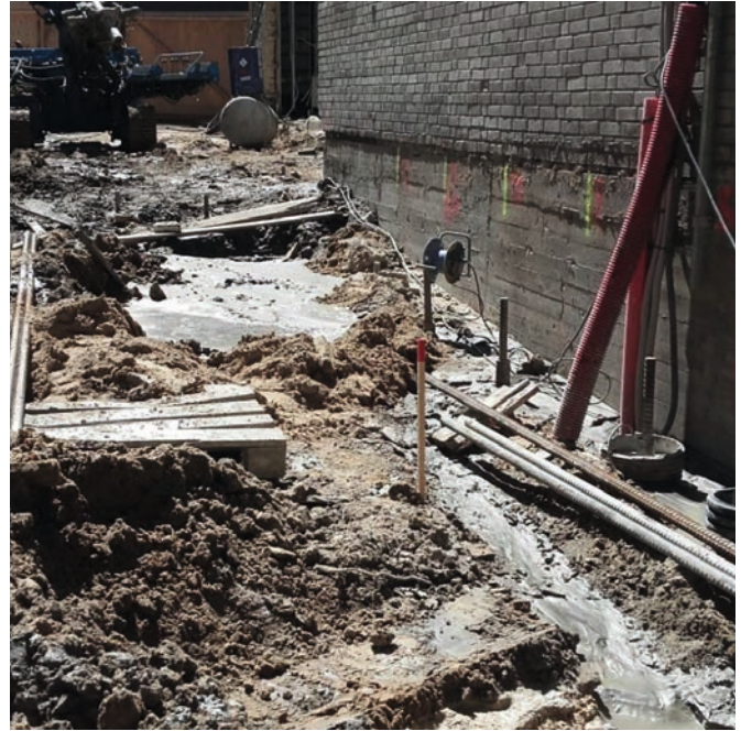
Image 3: Plastic pipes as a drill guide and conditions on building site
