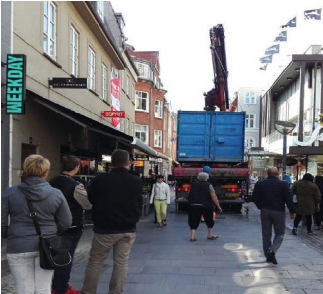
Image 1: Access to the building site in the pedestrian area
