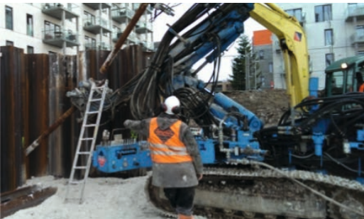
Image 1: Drilling activities in limestone using overburden drilling technique
