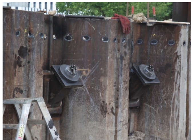
Image 2: Pre-tensioned line anchors prior to installation of the steel caps.
